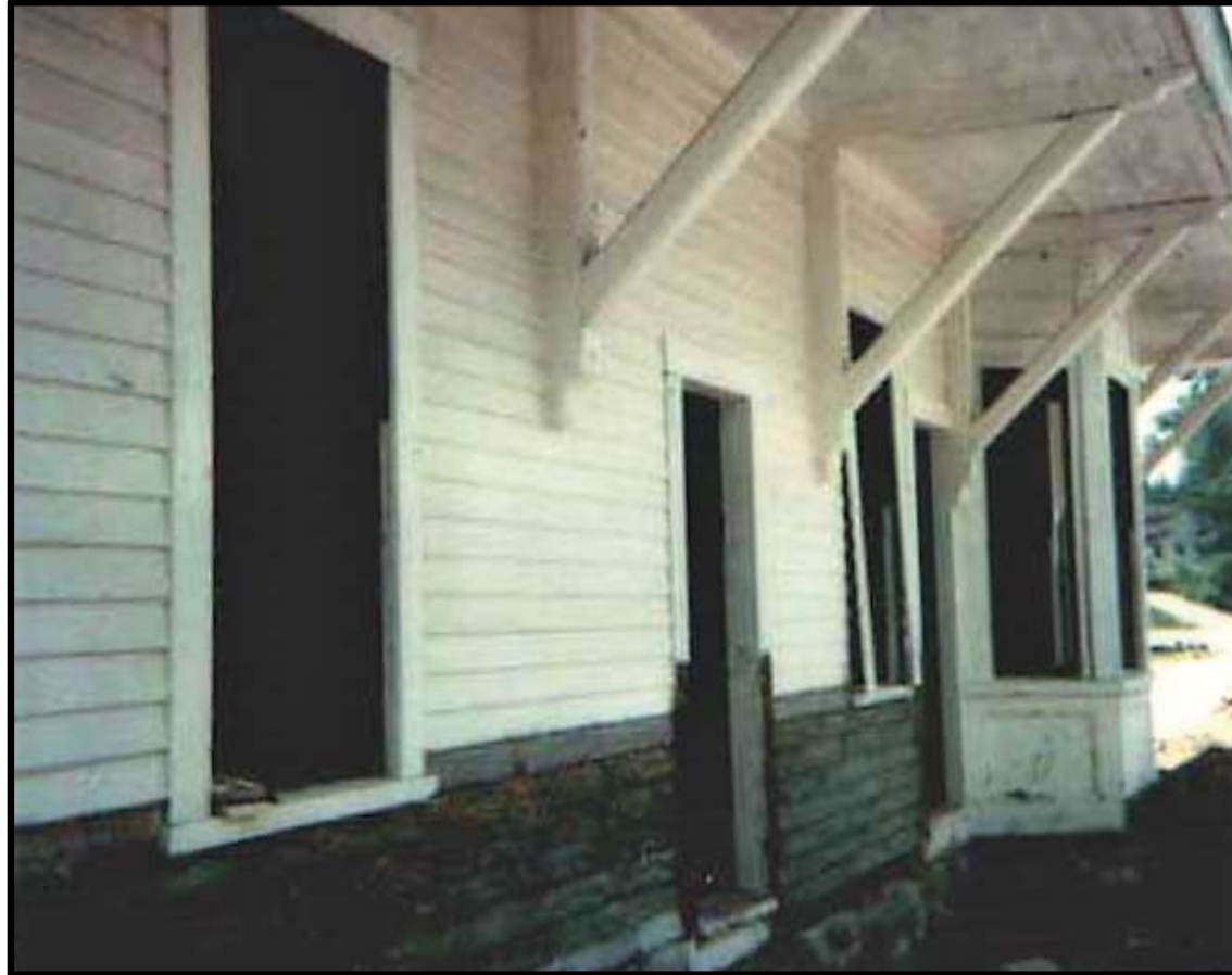
Image Number 12 North trackside elevation of the building circa 1977.
