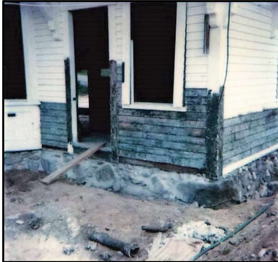
Image Number 14 Northwest corner foundation detail circa 1977.
